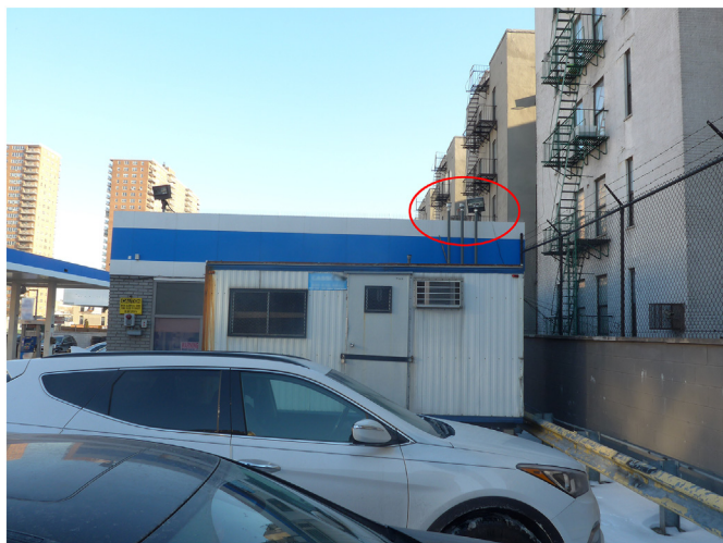
Fig. 1. The three vent pipes (enclosed by the red ellipse) on the right side of the convenience store of a gas station are <10 m away from the residential building.
